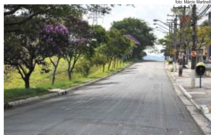
As obras de recapeamento na Avenida Yojiro Takaoka
